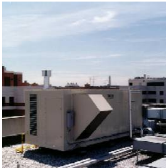
Fig. 8. A Desiccant Unit Atop the Park Hyatt Hotel, Washington D.C. (Source: National Renewable Energy Laboratory, DOE)
